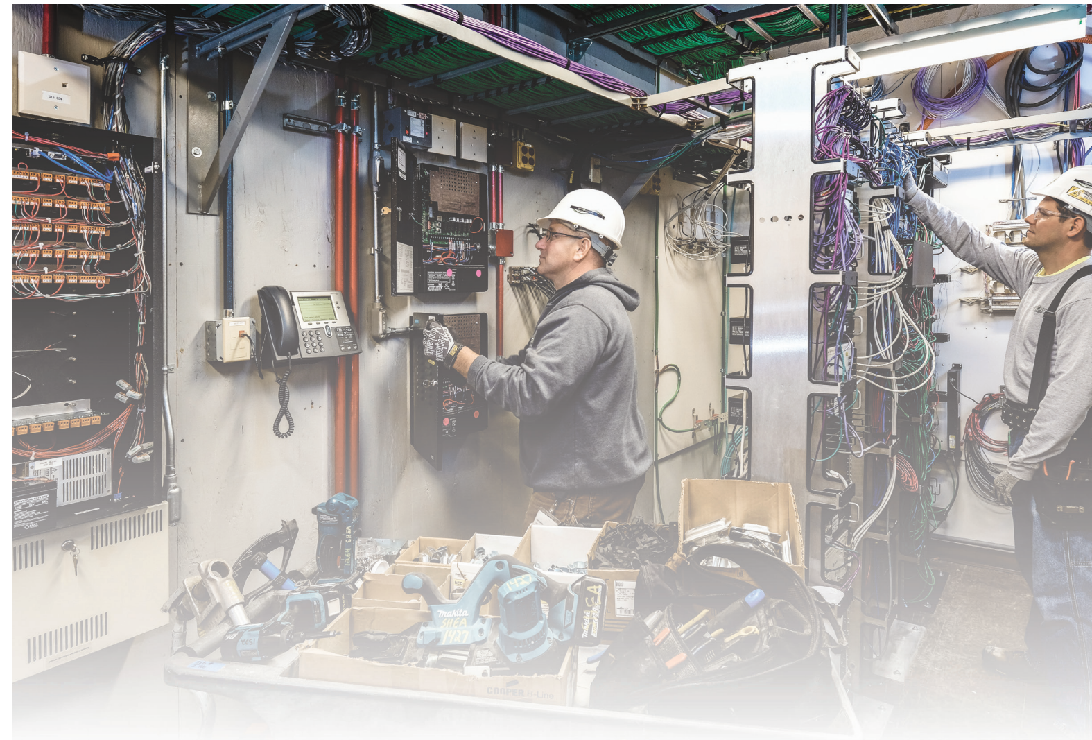
Photo Above taken by Weston Imaging: Shea Electric's Roger Martel and Shane Wall work in a telecom closet (IDF)
